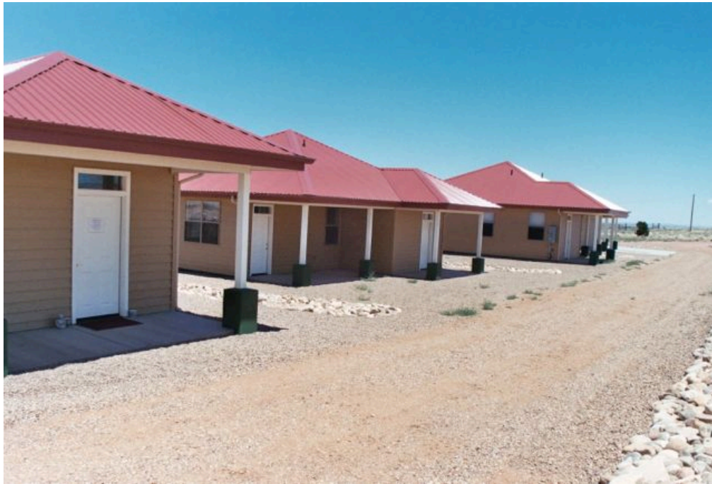
The four rental houses built by the state of Arizona.
