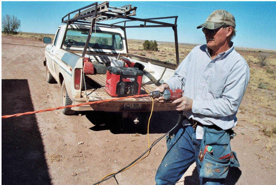
Twisting ROMEX cable, using a power drill
