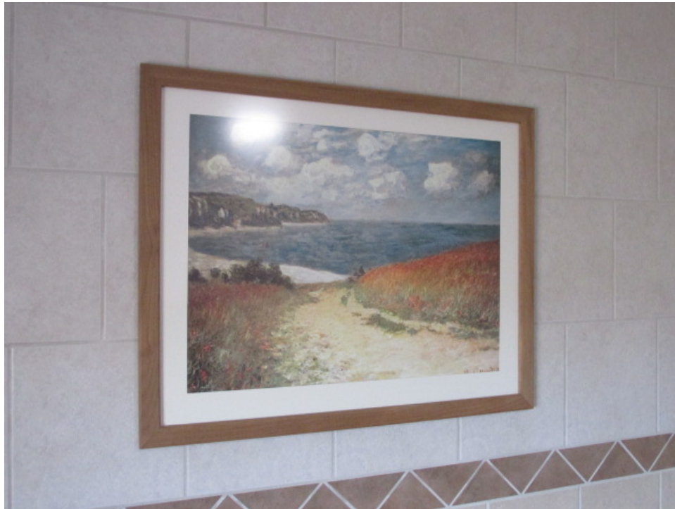
Nails can transfer microwaves through the shielded walls. Pictures are instead hung using self-adhesive fasteners.
