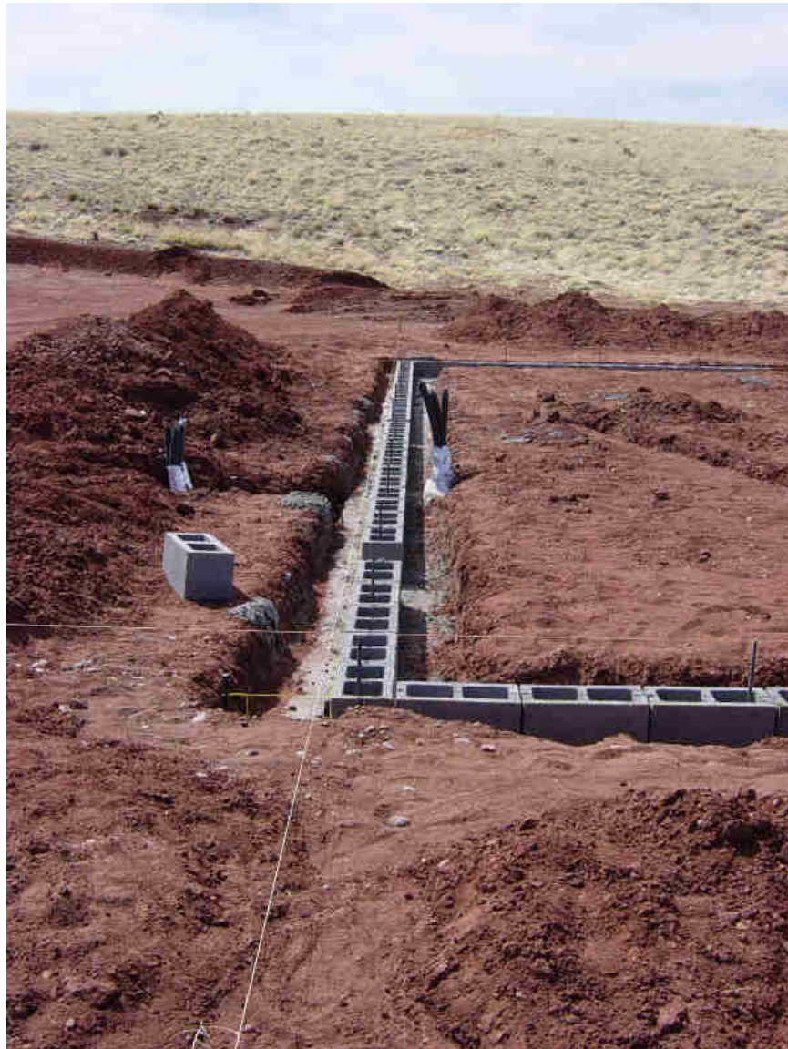
The start of the stem walls, with steel rebar reinforcement. These rebars were not connected to the grounding system.
