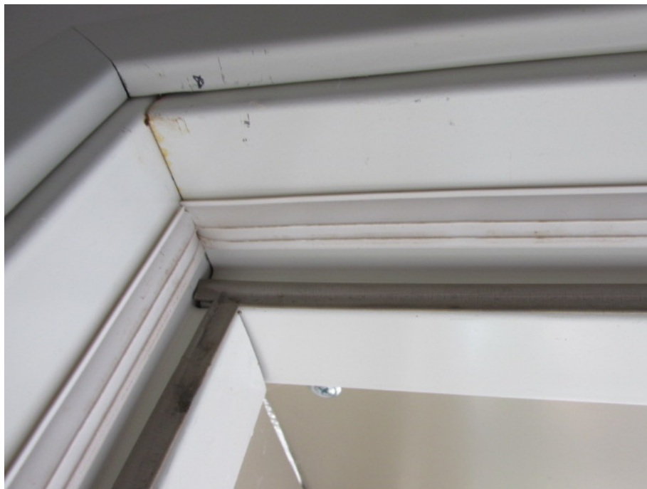
The steel frame of the front door with conductive gaskets that seal the air gap between the door and the frame.
