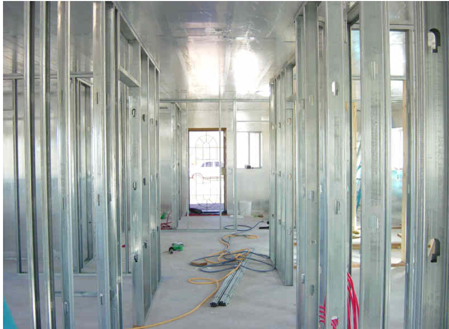
The interior walls were framed with steel studs after the exterior walls were walled in and covered with aluminum foil.
