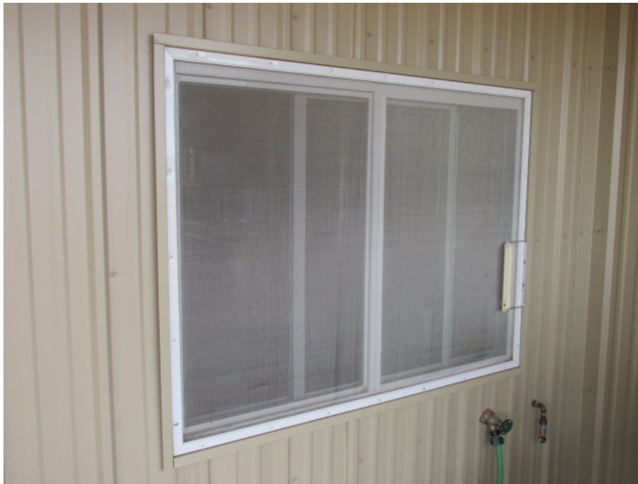
The finished window with stainless steel mesh screen, after the steel siding was installed.
