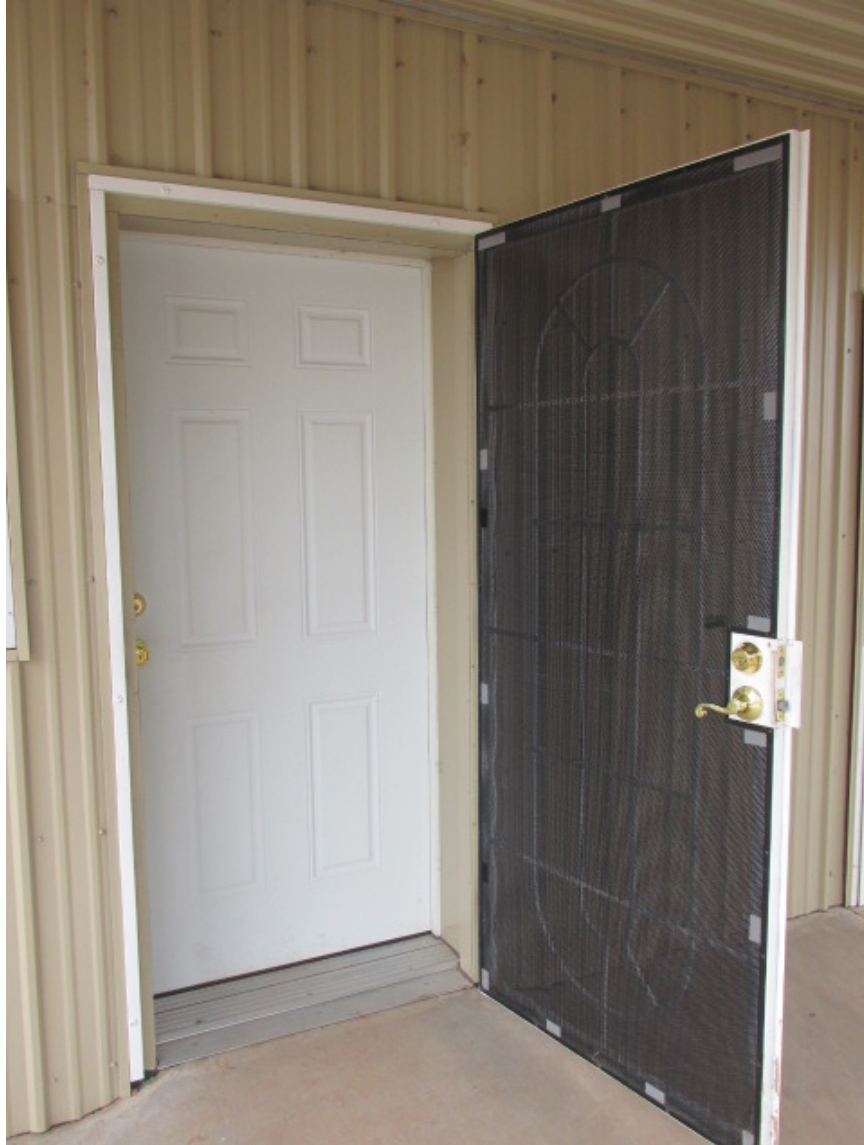
The front door is of steel, with a steel frame and a steel-mesh screen door.
