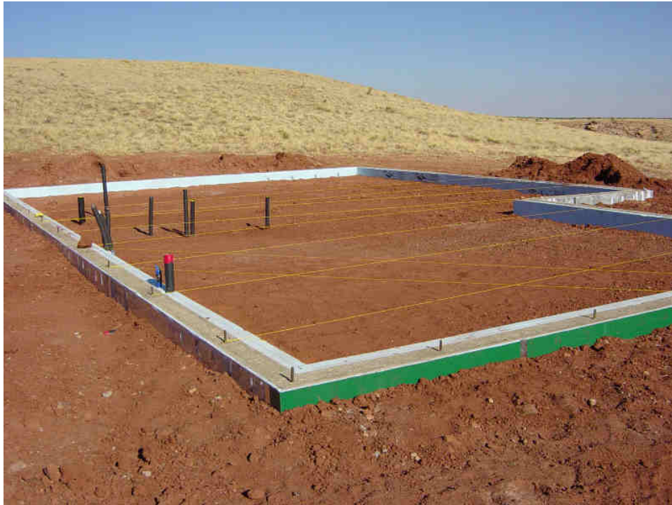
The outside of the stem wall is shielded with galvanized steel plates. They used recycled steel plates, some of which happened to be green.
