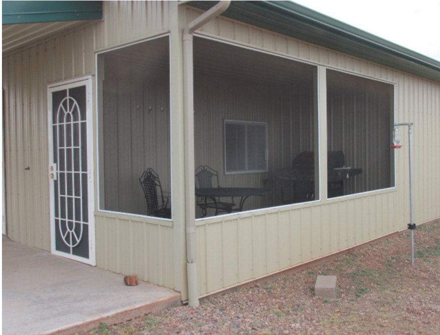
The porch is outside the house shielding, but still reduces the microwaves about a hundredfold (20 dB).
