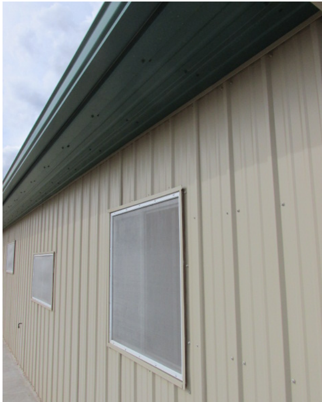
The soffits are a part of the outer shield and made of steel siding. The slit between the soffit and the wall is shielded with metallized plastic (hidden behind the soffit-siding connection.)
