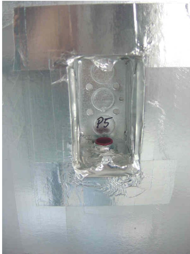
Electric box sealed to the foiled wall with aluminum tape. The backside was also taped to seal the slits around each knockout.
