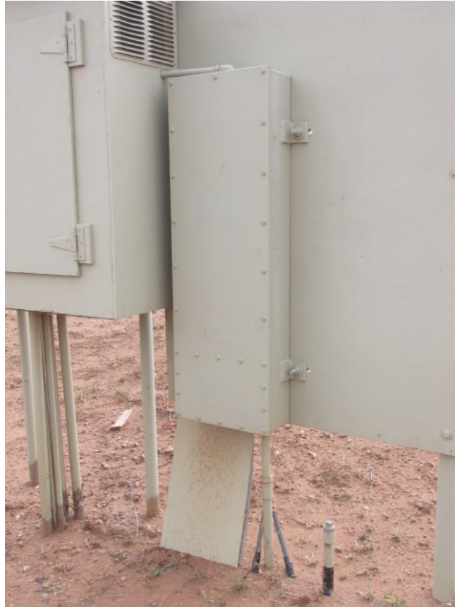
Heavy-duty filter on the electrical feed for the house. Note the metal casing and conduits that prevent the wires from picking up microwaves from ambient radiation. There is also a wide grounding strap.
