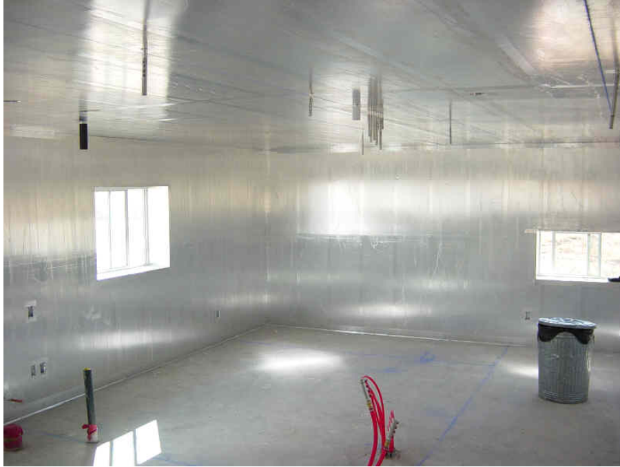
The inside shield was applied to the finished exterior walls before any of the interior walls were framed.
