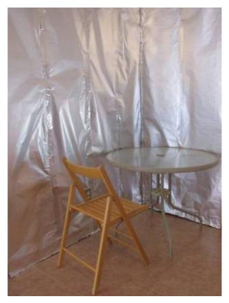
Room shielded with foil from a grocery store. The floor needed no shielding.
