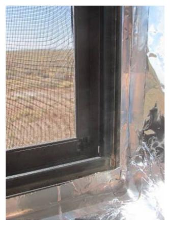
With low-E glass the window is already shielded, though foil must be installed to cover the frame, sill and the rest of the window hole. This window has an insect screen that does not provide any shielding.
