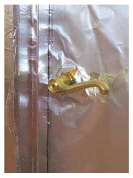
The shield must go snugly around the door handle. The door frame should also be shielded.
