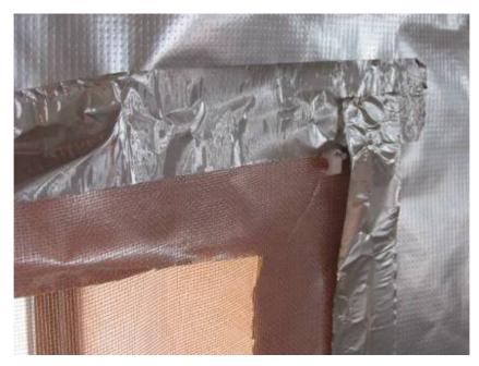
Copper mesh shields the window on the inside. The mesh is mounted onto the aluminum shielding using a couple of nails and lots of aluminum tape.
