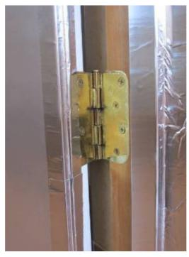
The foil is attached with aluminum tape all around the door edge. The room side of the frame is shielded with aluminum tape.
