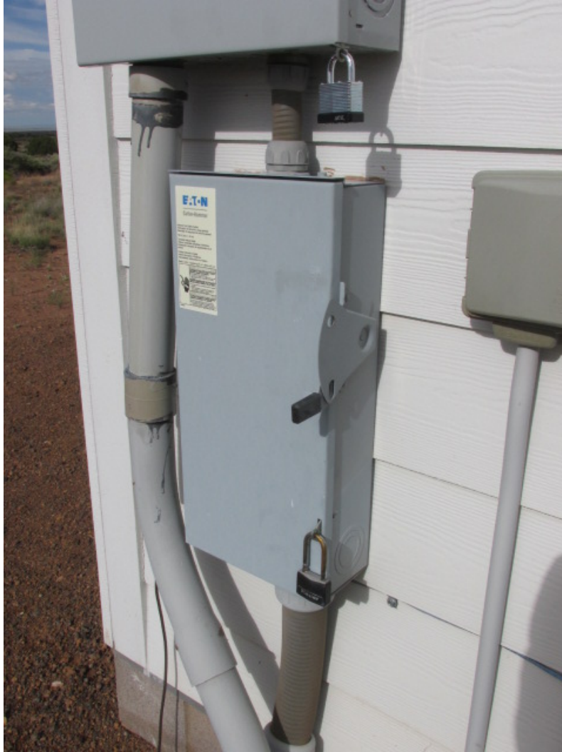
Three-poled whole-house kill switch to disconnect the two phases and the neutral to a home in the USA. In areas served by three phases (most of Europe), a four-poled switch is needed. This box is mounted below the master panel on an outbuilding.
