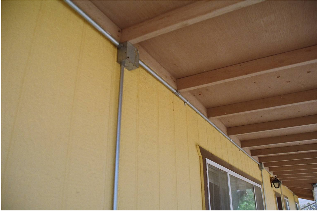
Metal conduits mounted on the outside wall, under a porch roof, since it was not possible to install them inside the existing wall.
