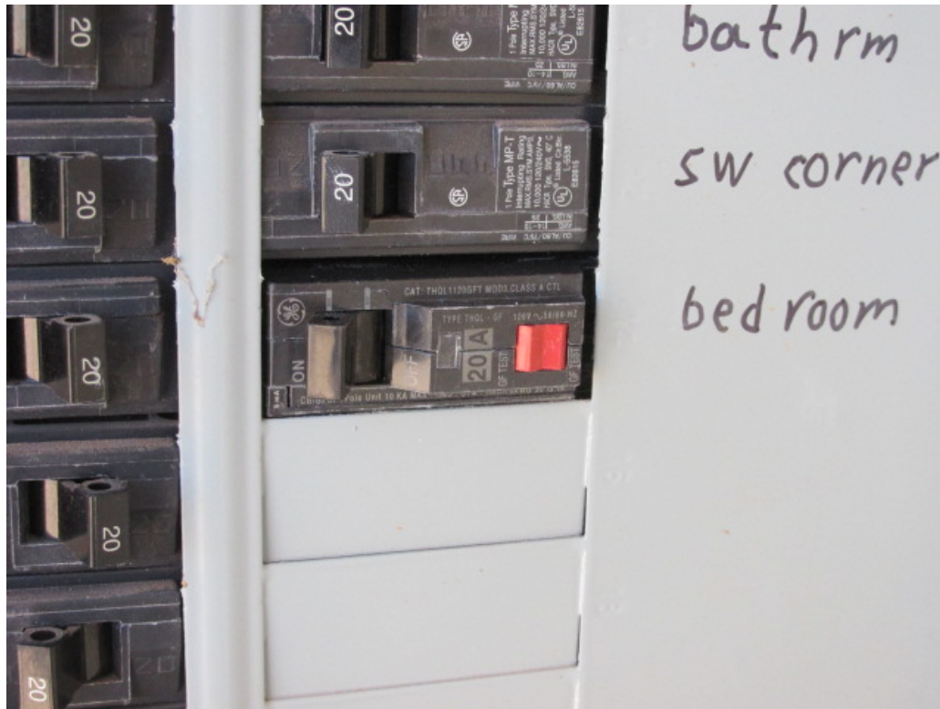
AFCI breaker in a breaker panel. It serves the bedroom and can be recognized by the red test button.
