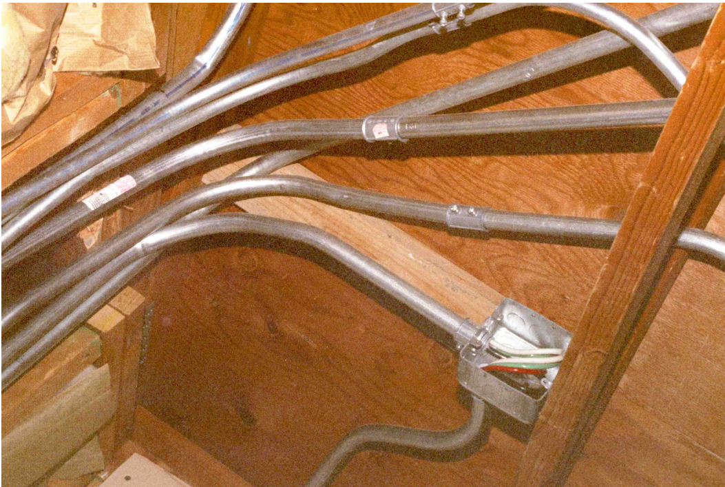
Metal conduits spreading out across the ceiling near the breaker panel in a house.
