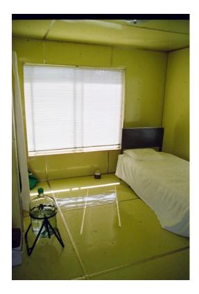
The camp has a variety of structures, which all are based on the porcelain-on-steel panels that were often used in MCS housing during the 1980s. These plates are expensive to buy and difficult to work with, as they must first be cut to the exact size and then shipped off to be covered with the ceramic coating. This process can only be done in specialized facilities and involves baking the plates in a large oven. These plates are rarely used today.
