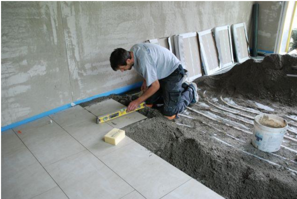
Installing the floor tiles with thickset mortar.
