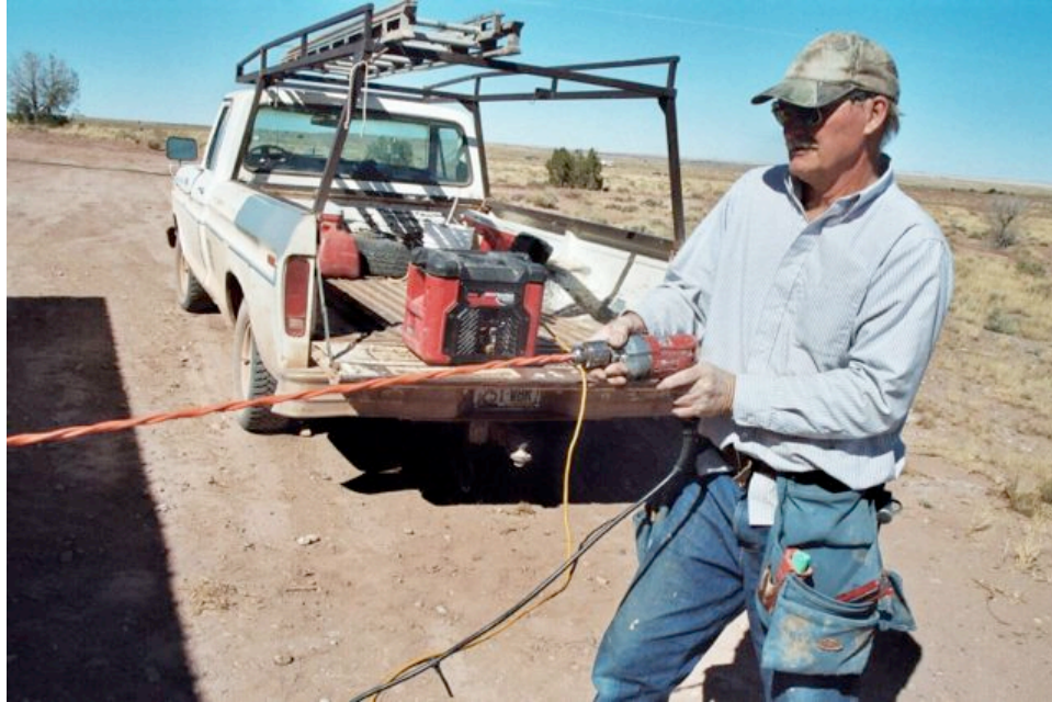
The contractor twisting the wires, using a power drill.
