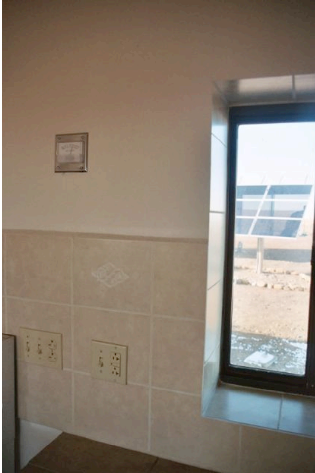
Analog voltmeter on kitchen wall, where it is easy to glance at it.
