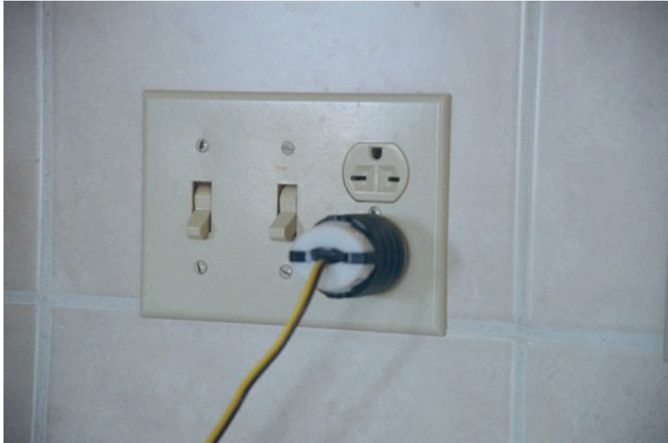
12 volt light switches and outlet. The left prong is plus, the right is minus.
