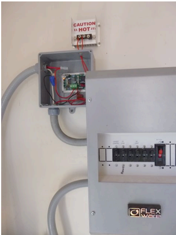
Voltage controlled switch (active high) from Solar Converters Inc., with a blocking diode on top and breaker box to the right.
