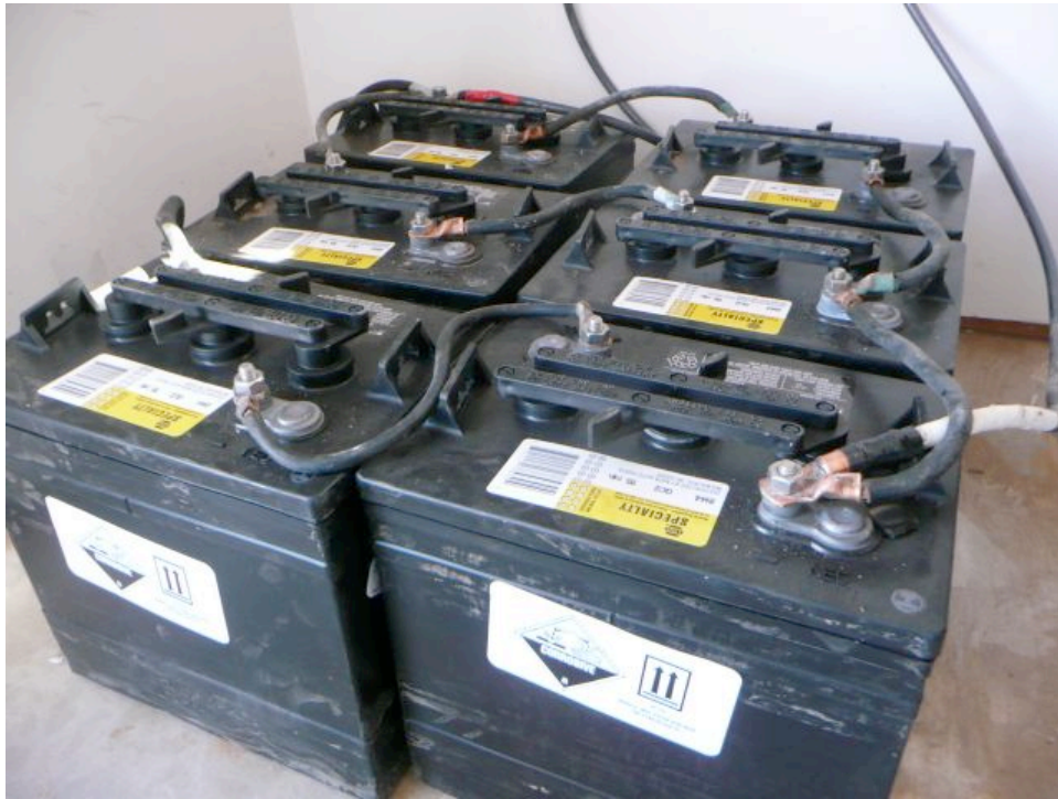
The main battery bank with six low-cost golf cart batteries.
