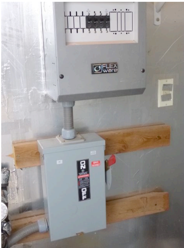
Main house breaker panel (top) and two-poled disconnect (bottom), which is located in utility closet on the side of the house.
