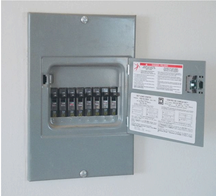
Breaker panel from Square D's QO series, which can be used for either AC or low-voltage DC electricity.
