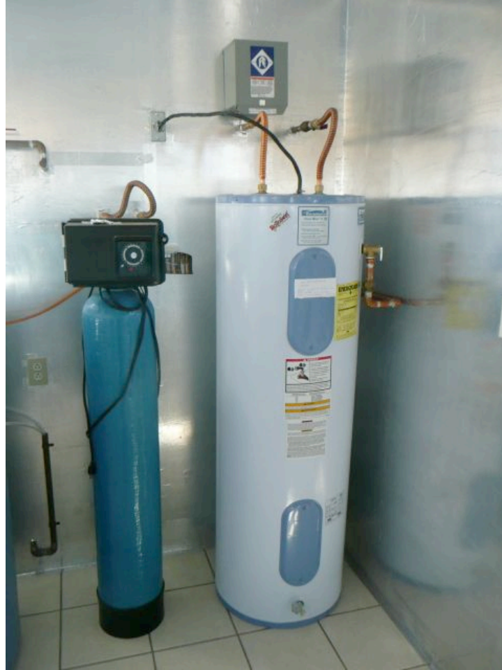
The electric water heater (right) is in the corner of the house, right next to the electrical panel (on the outside) to minimize radiation. The blue iron filter is on the left.
