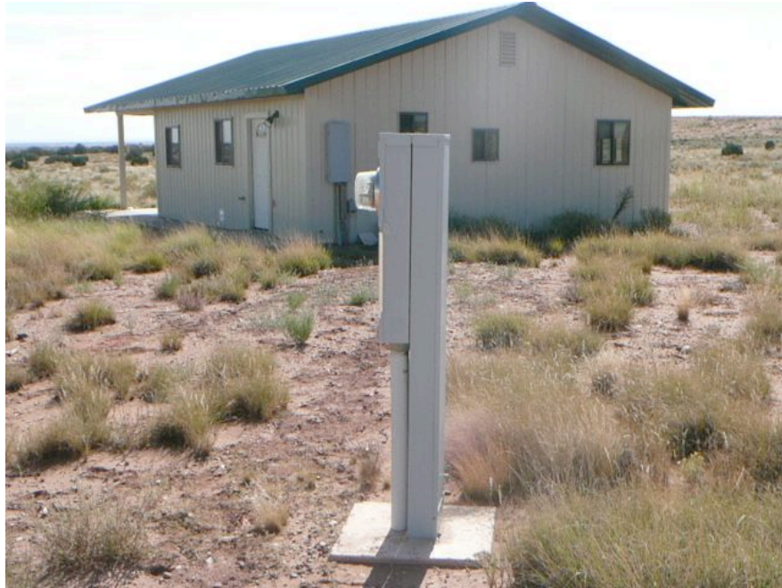
The electrical meter is placed on a pedestal away from the house, to minimize EMF.
