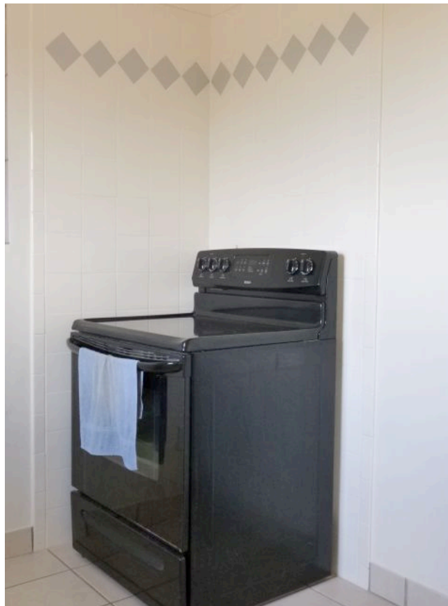
The cooking area has tiles on the wall to protect the clay paint against splashes.
