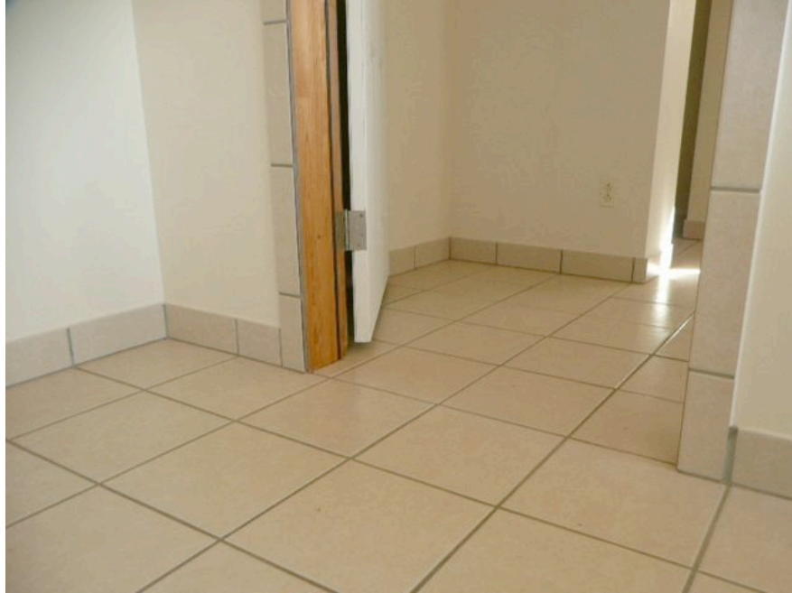
The floors are all tiled. Tile is also used for the baseboard and the trim around the doors.
