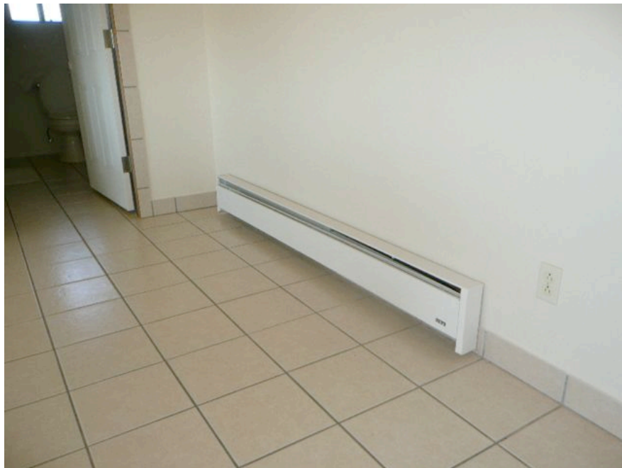
Low-EMF electric baseboard heaters are located to minimize EMF exposures. The owner does not use the bedroom heater while sleeping.
