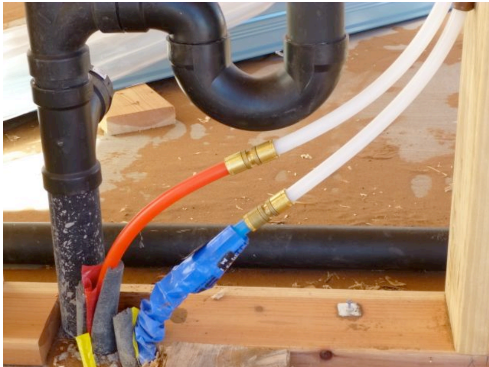
PEX crimp connections, before the wall was closed in.
