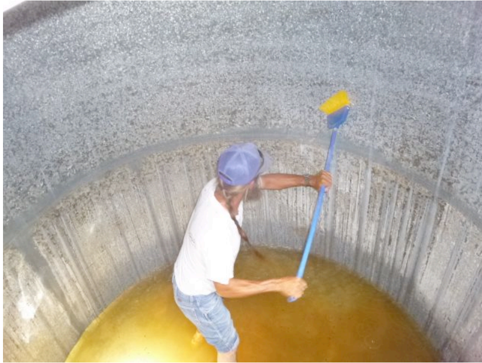
Cleaning the inside of a 3000 gallon (11,000 liter) steel water tank.
