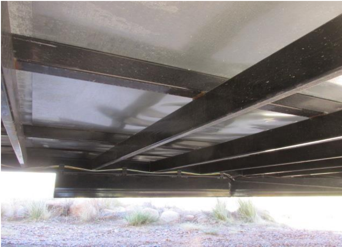
The floor is all steel, no plywood at all.
