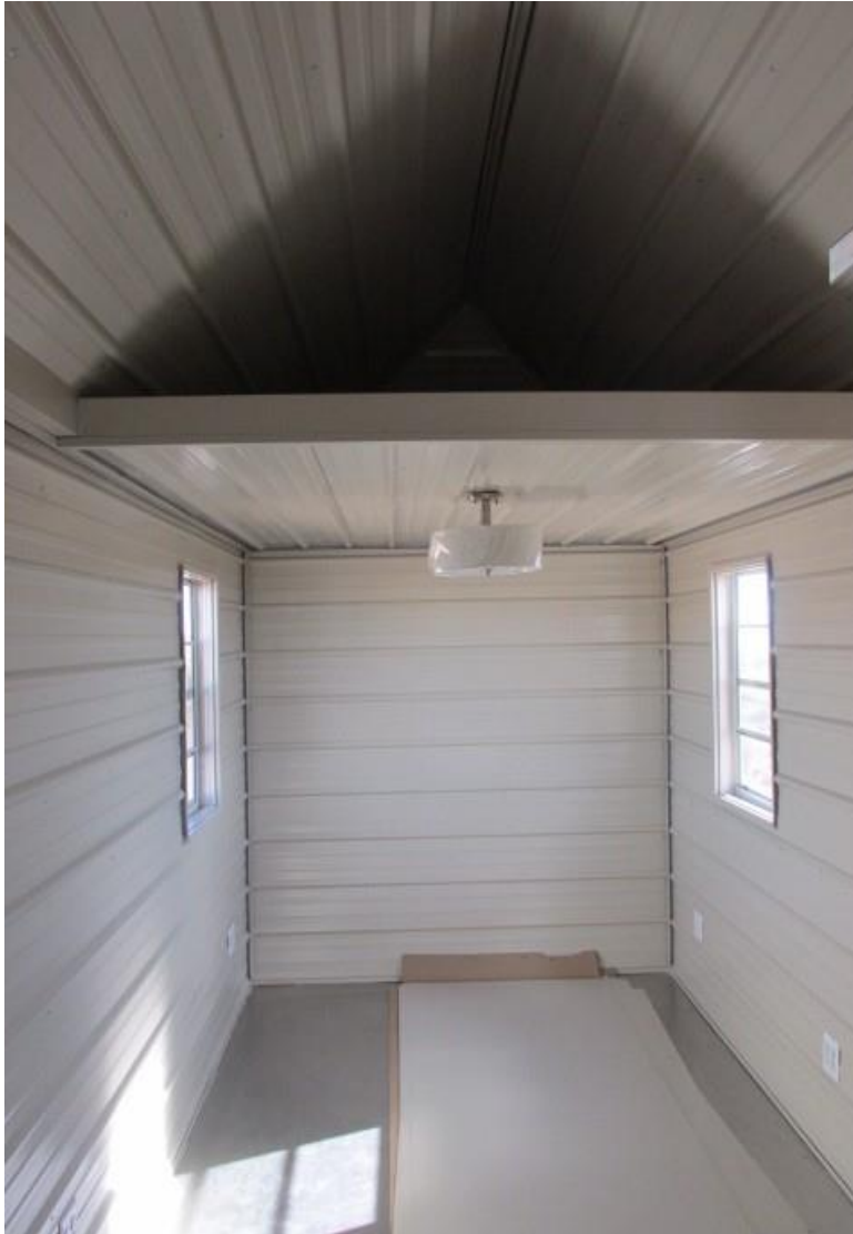
A small loft covers half the length of the house. The floor is stainless steel.
