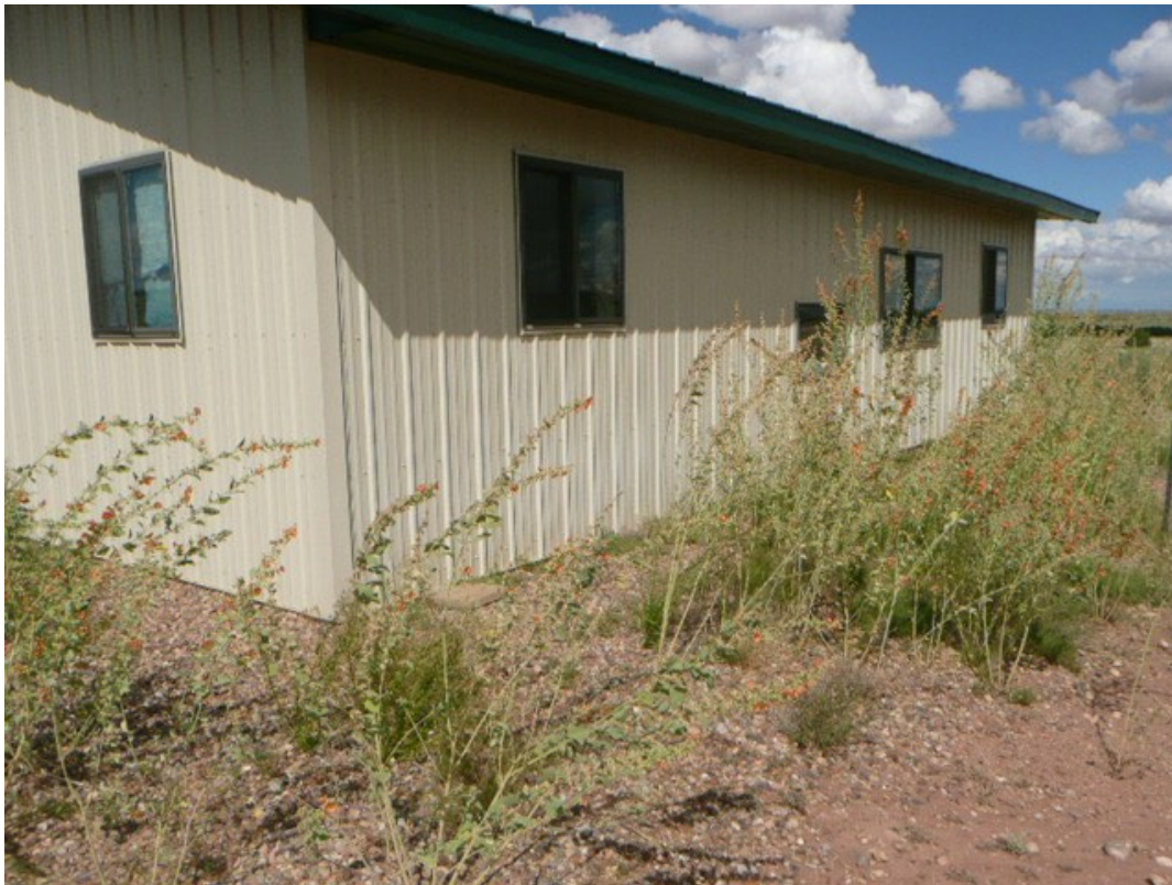
The outside of House-3, with steel siding, steel roof and metal-coated low-E windows.
