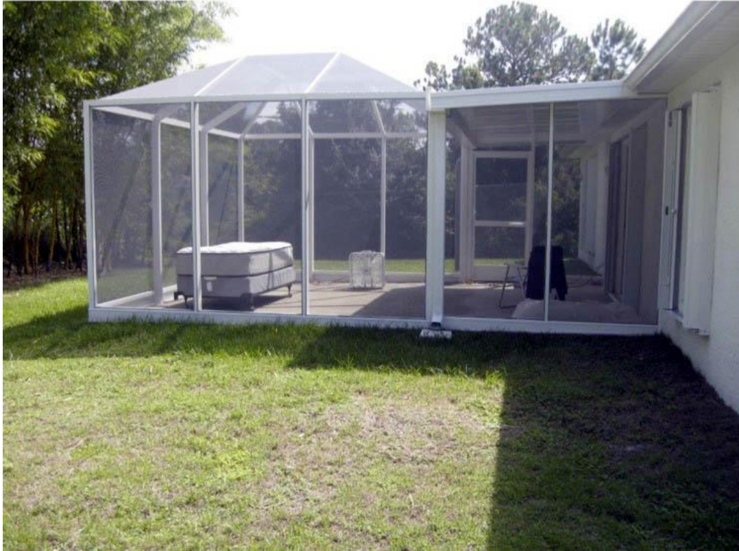
This shelter was built in Florida in 2014, using materials for screened porches. It is attached to the porch of the house. Picture courtesy of Nathalie D.
