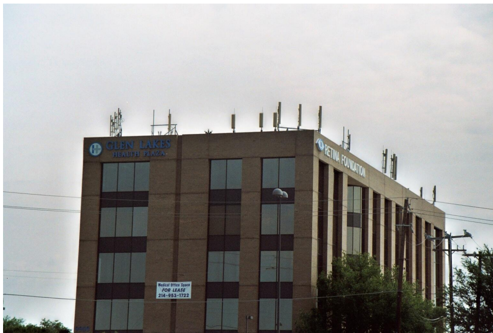
Office building with several cellular base stations on the roof.
