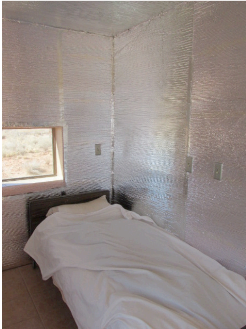
Aluminum foil is cheap and effective shielding that can be installed in several ways.
