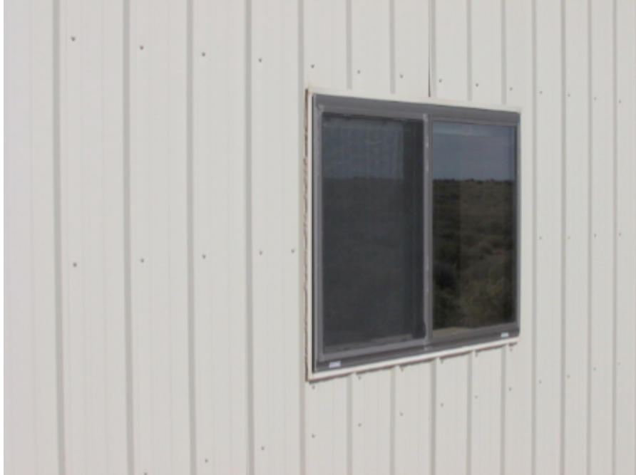
Steel siding and roofing are good shielding materials.
