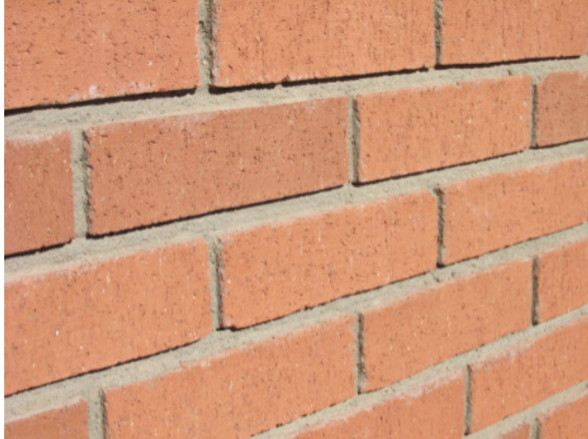
Walls of brick or concrete absorb microwaves, but rarely enough to provide good shielding.
