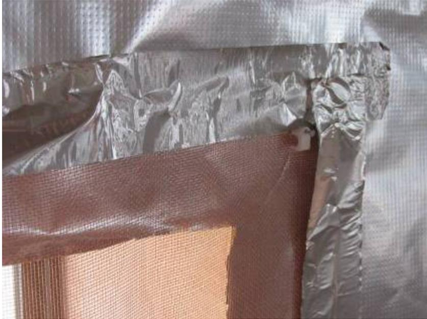
*Copper mesh shields the window on the inside.
