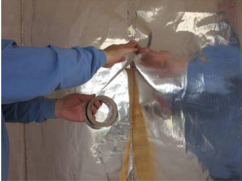
*Taping the seam*
