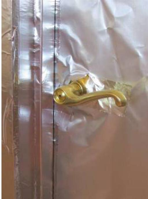
*The shield must go snugly around the door handle.
