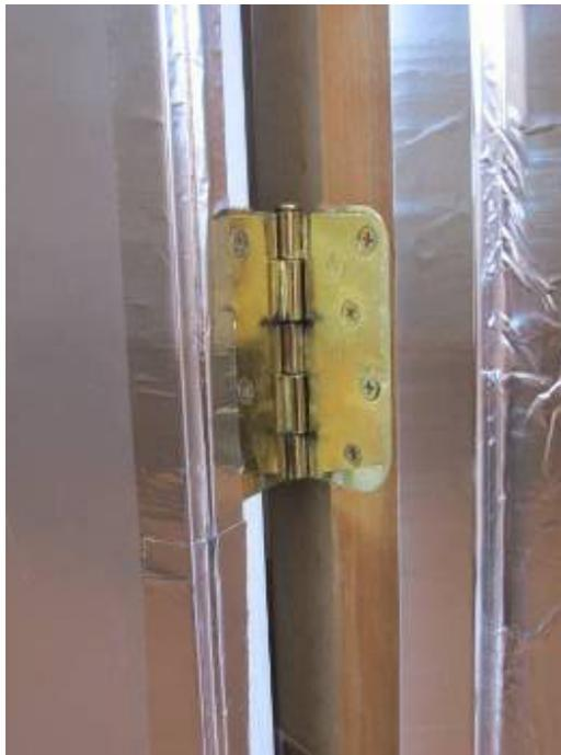
*The foil is attached with aluminum tape all around the door edge.
