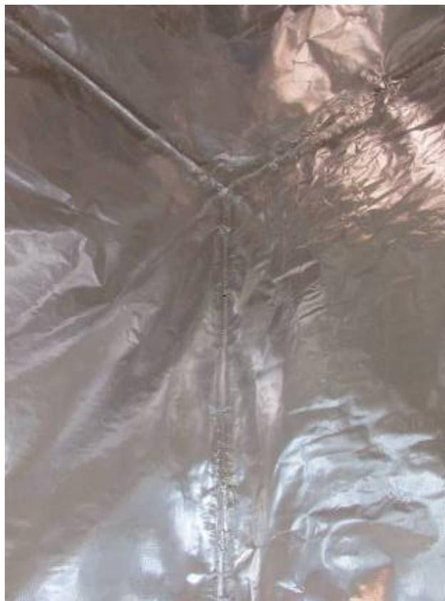
*Seal all seams between walls and ceiling with aluminum tape.*
