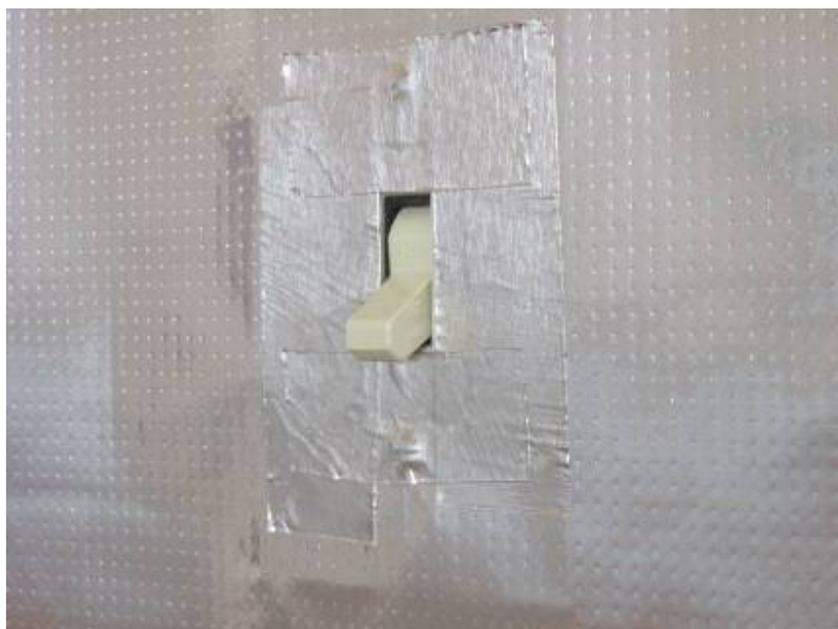
*Then tape closely around the switch to maintain the shield.*
