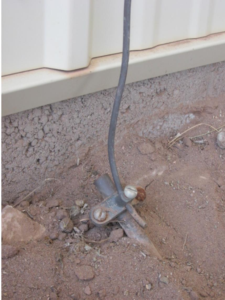
*The ground rod is usually located right below the main electrical panel, with a wire connecting the two.*
