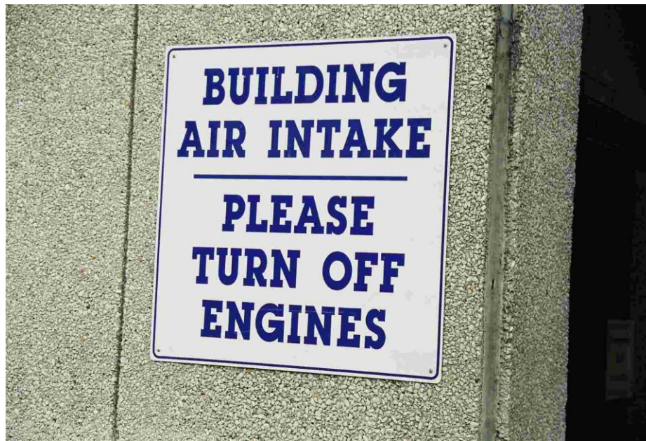
The air intake to many office buildings does not provide clean air because of poor location at street level.
