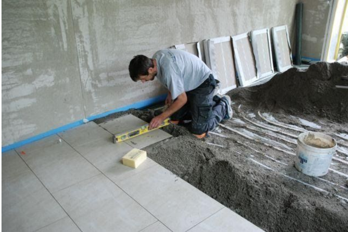
Installing the floor tiles with thickset mortar.
