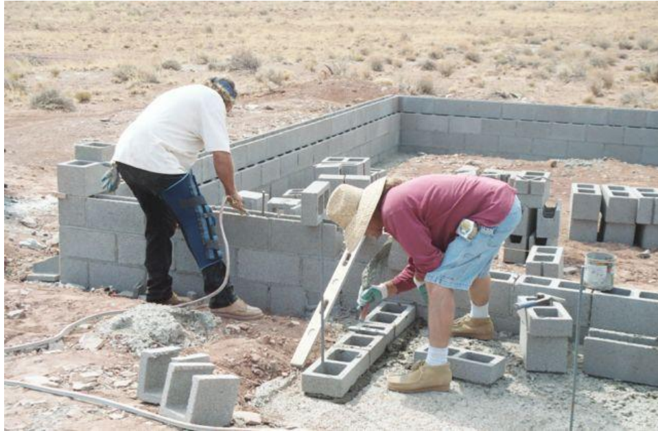
Building the stem wall.
