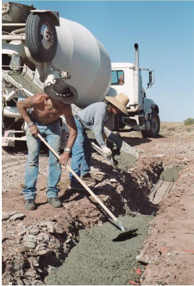
Pouring the footings for the stem wall.
