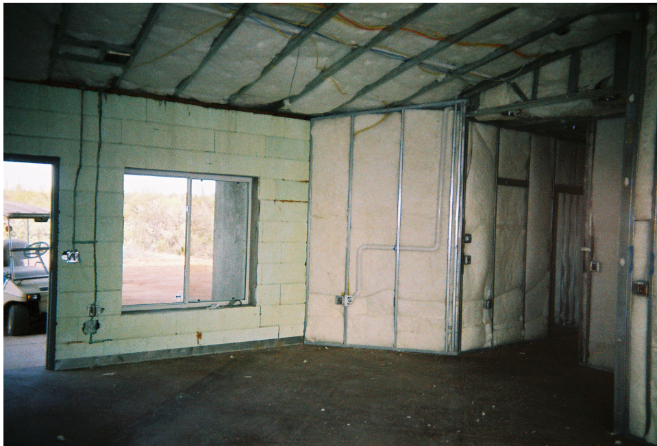
The walls and ceilings were insulated with formaldehyde-free fiberglass.
