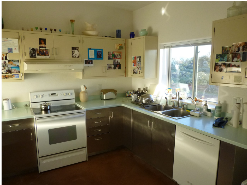
The upper kitchen cabinets are of powder-coated steel, while the lower cabinets are stainless steel.
