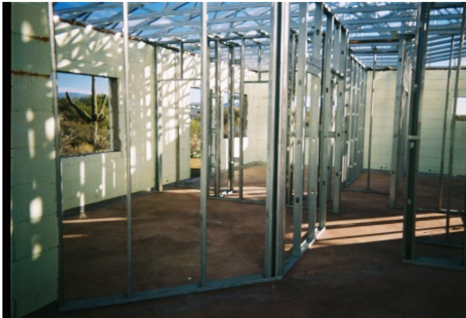
The interior walls were made of steel studs that were degreased.
