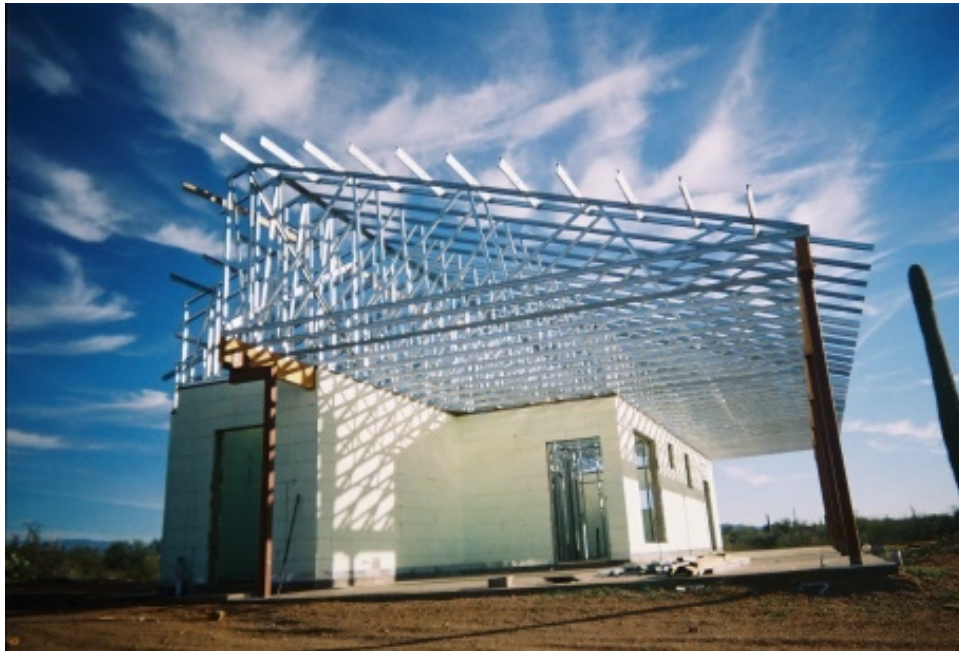
The steel trusses.
