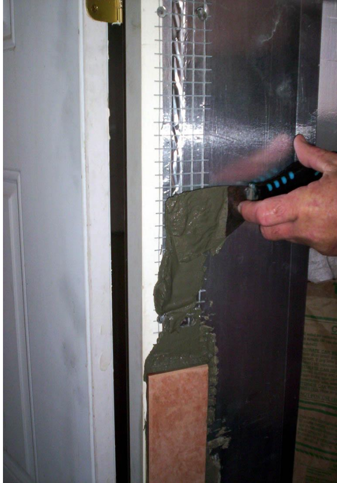
Spackling thinset on the steel hardware cloth.
