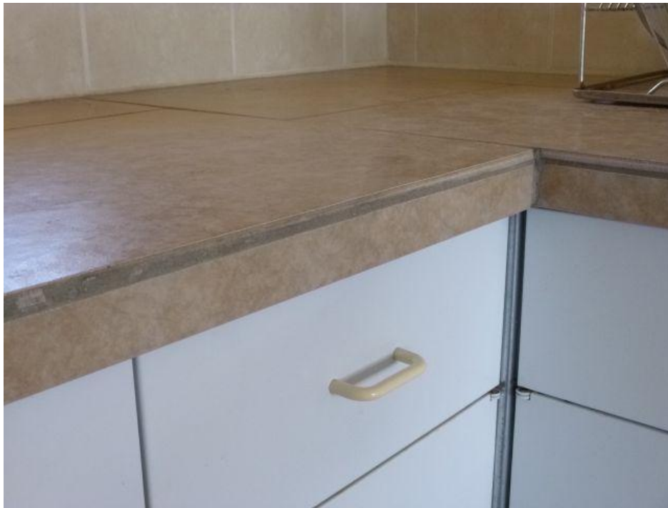
Detail of tiled kitchen counter; with three layers of HardiBacker cement boards underneath.
