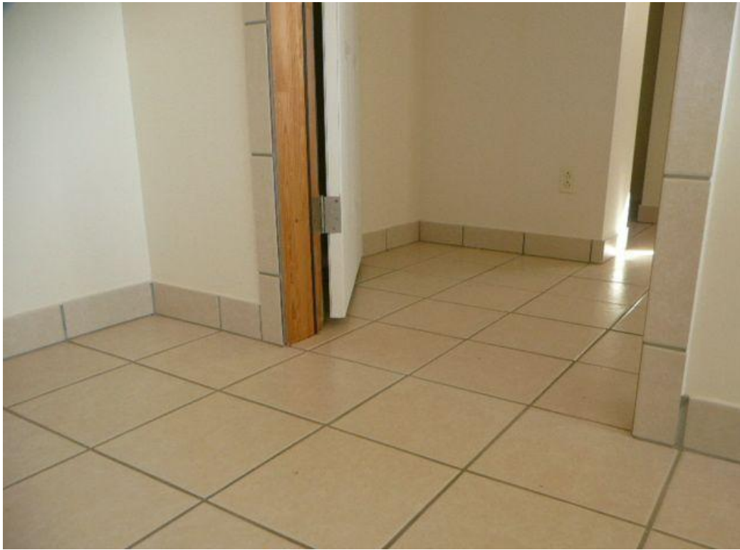
Tile used as floor covering, baseboard and trim around the door
