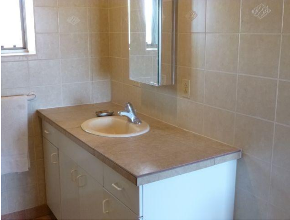
Bathroom cabinet with tiled counter on top of HardiBacker cement boards.
