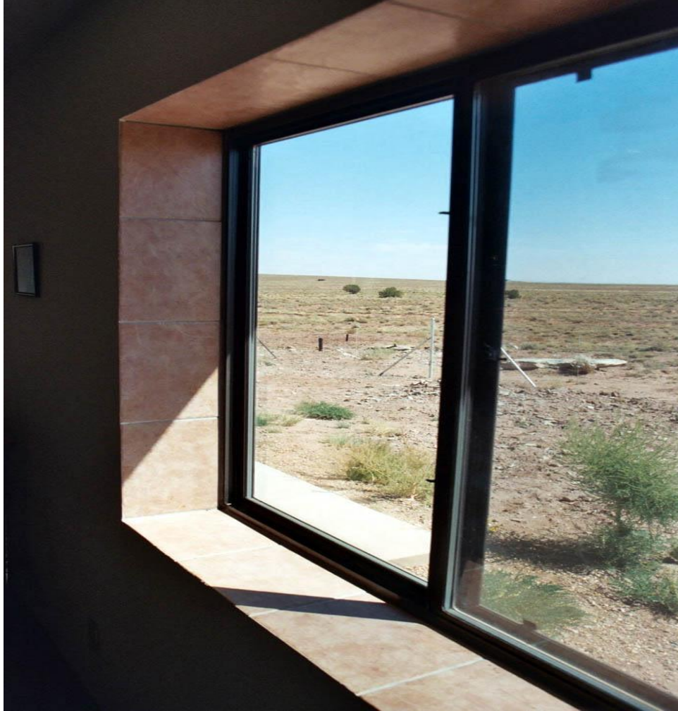
Tile work around a window, with HardiBacker cement board underneath.
