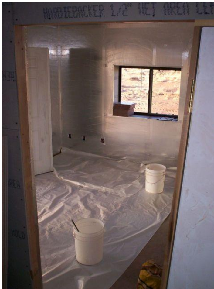
Wet curing floor tiles under plastic sheeting.
