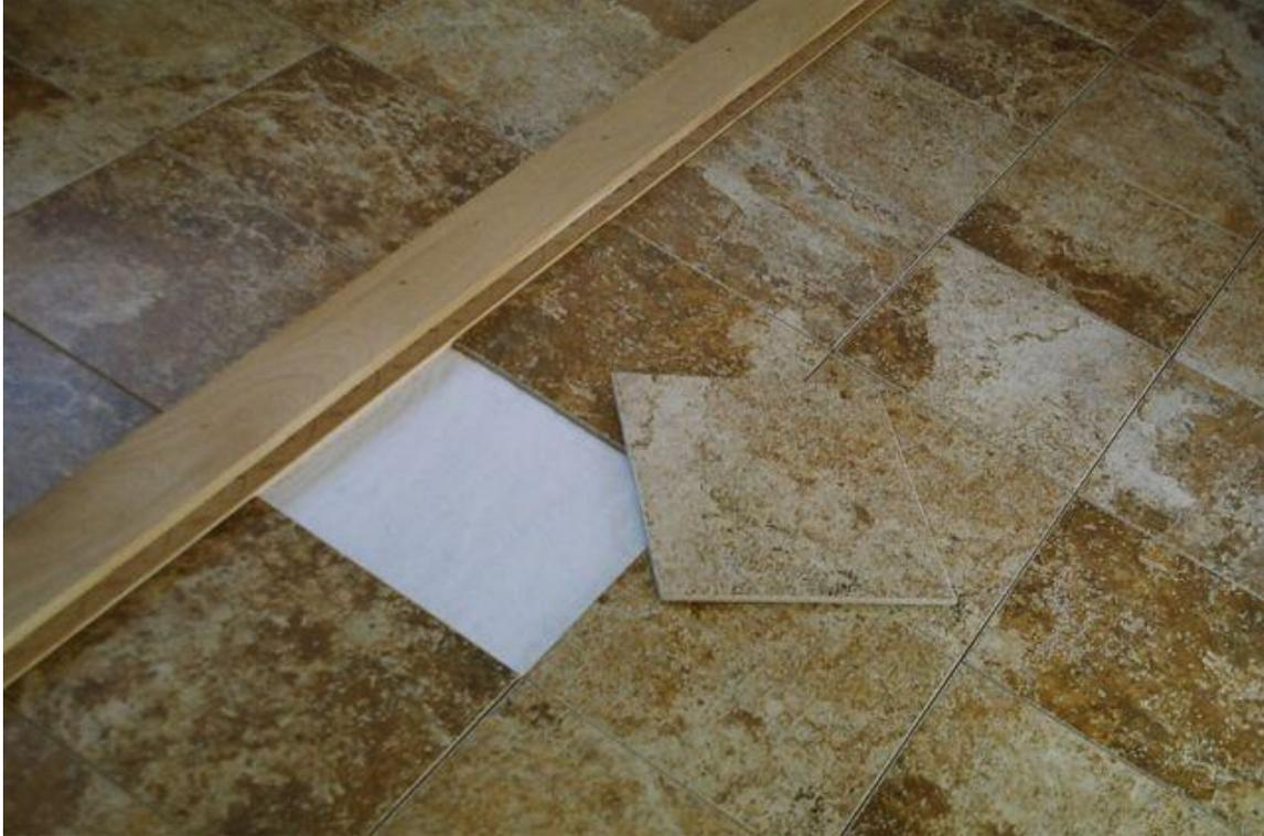
*The carpet was replaced with loose porcelain tiles on top of Tu-Tuff (polyethylene) plastic.*
