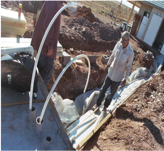
The heat tunnel between the house and outbuilding.
