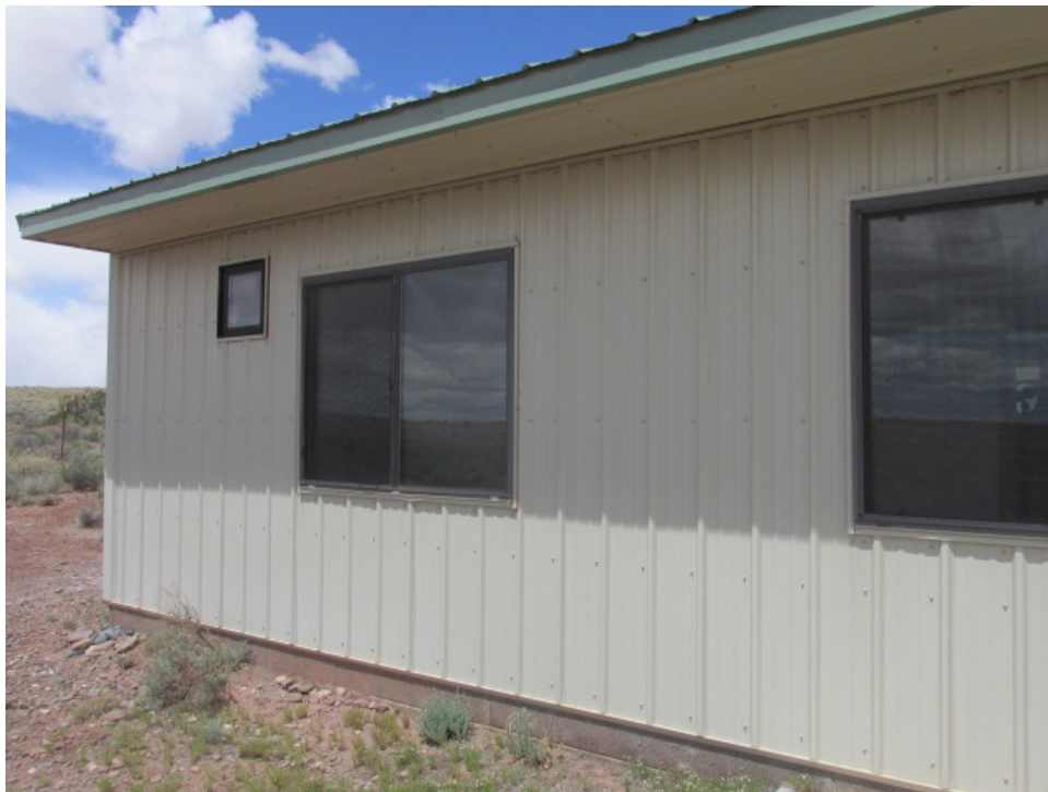
The roof overhang keeps the sun out during the summer and lets it in during the winter.
