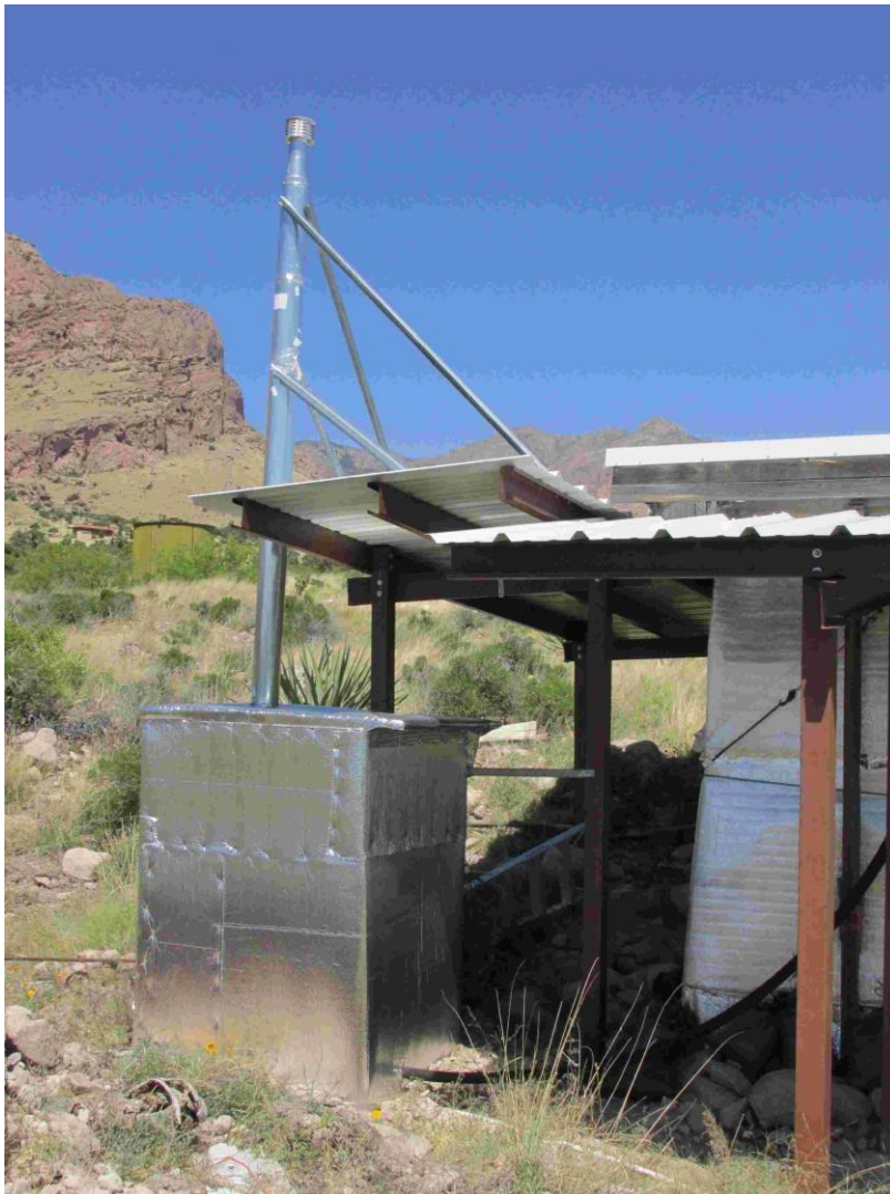
Outdoor propane water heater to heat the cabin, which by then also had sun shades and some insulation (2015)
